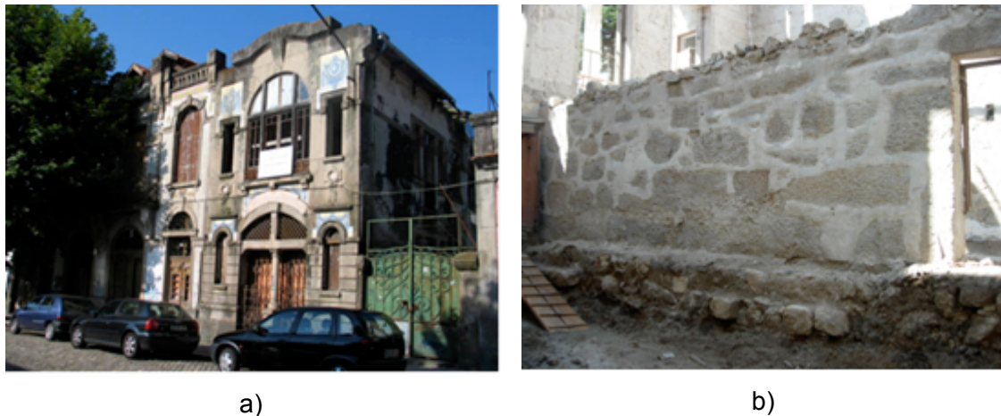
Figure 3: António Carneiro building: a) general view and b) the tested wall.
