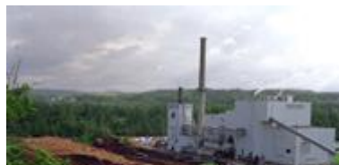
McNeil Generating Station, Burlington, Vermont, the country's only utility-owned and operated wood-fired power plant.
