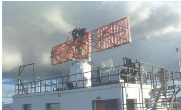
Figure N° 6: INVAP developed a secondary radar (a radar to detect commercial aircraft) and it is working on a primary surveillance radar (for military purposes and aircraft).
